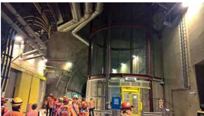
MFS Sedrun Lift (Foto: Björn Bauhofer)
